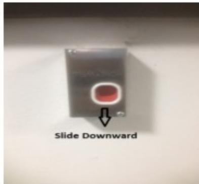
Insert your finger in the red button and slide **downward**, the red tab will protrude from the bottom portion of the panic button. The Panic Button has been activated.
